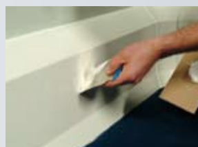
Damage to the Sanicoat can be easily and quickly repaired with the PolySto Repair Kit
